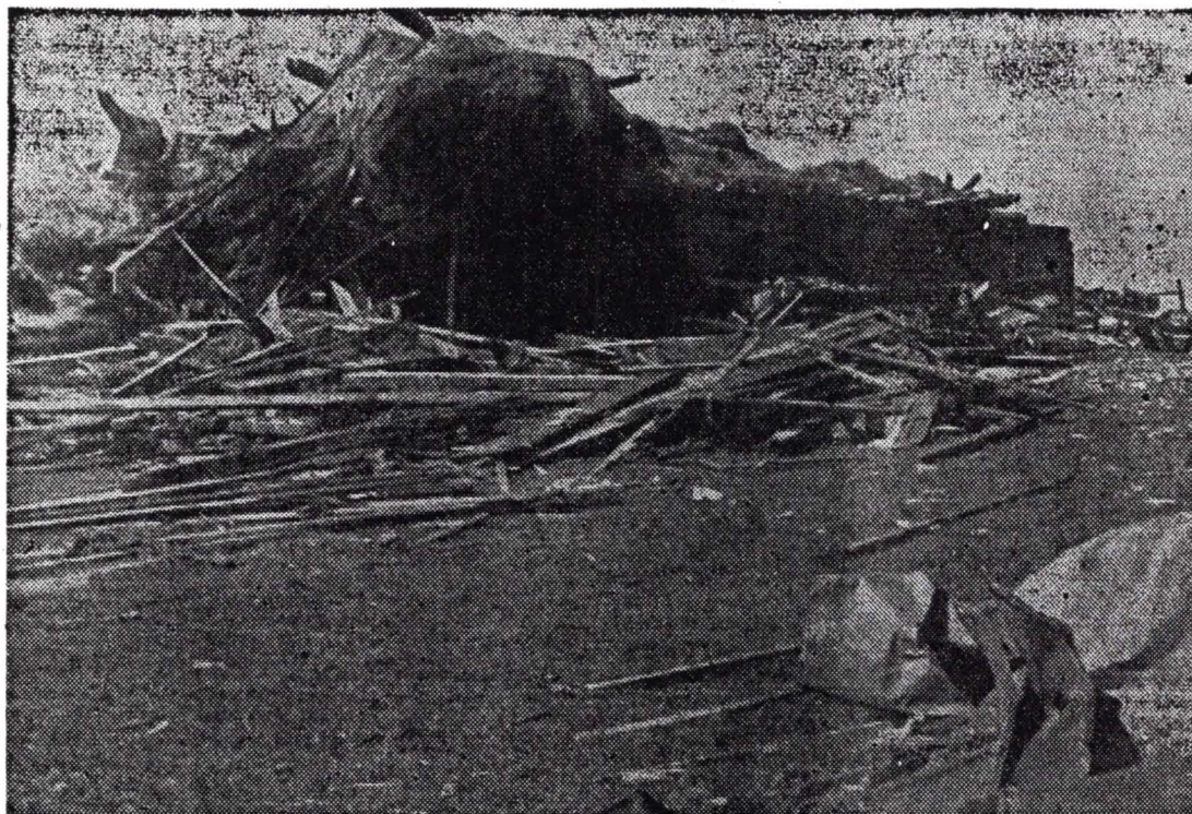
All that was left of the large frame barn on the Moore farm, south of Independence, after the recent cyclone had passed. This was one of the oldtime well-built structures in the county, put together with wooden pins.
