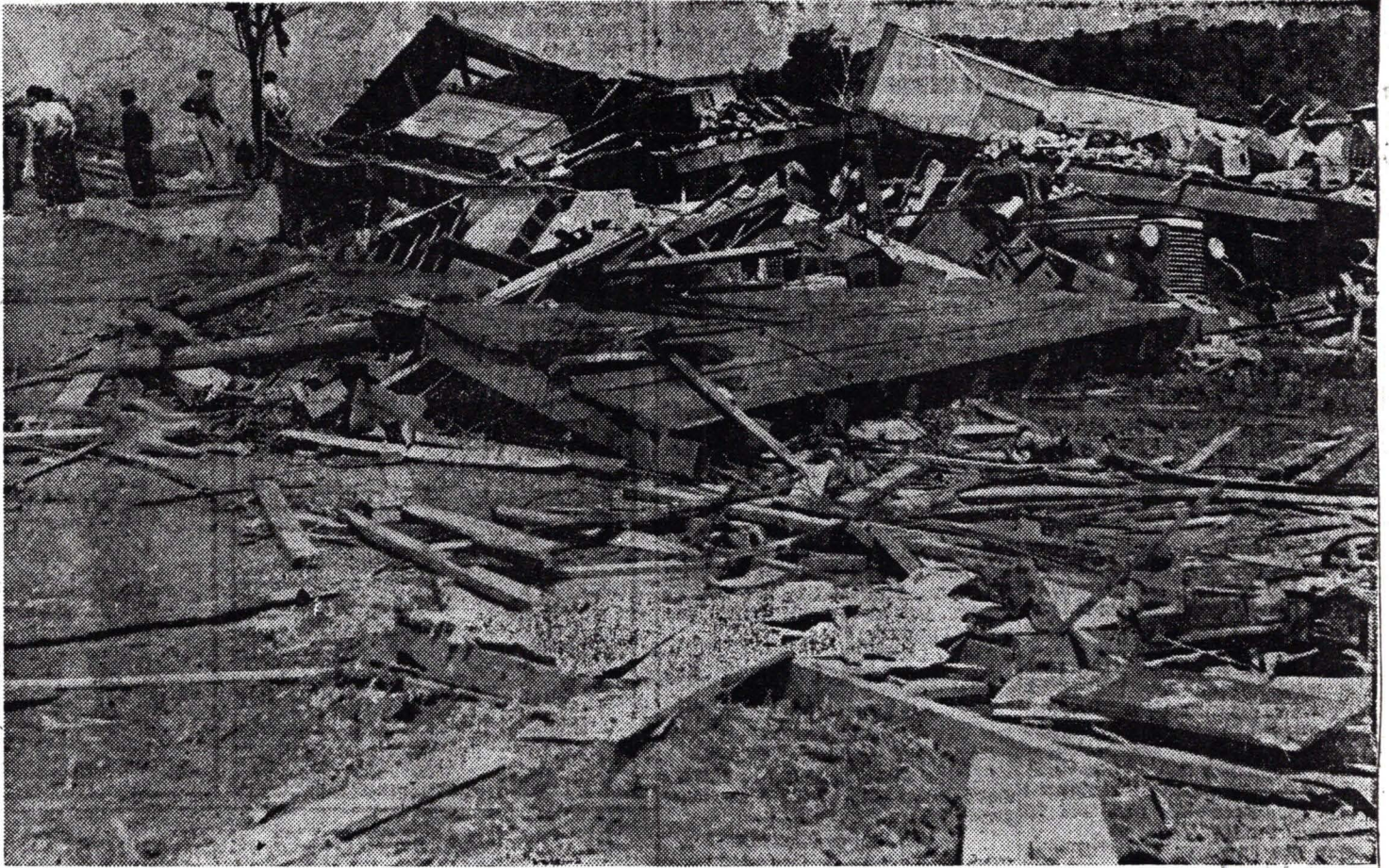
The company store, largest building in the Chartlers community, lies a mass of ripped, broken and tangled timbers, and much of the building material and stock is "gone with the wind." In the picture display cases are seen atop the tangled wreckage, and to the right is seen the nose of a truck caught and covered by the collapsed building. The building is a complete loss.
