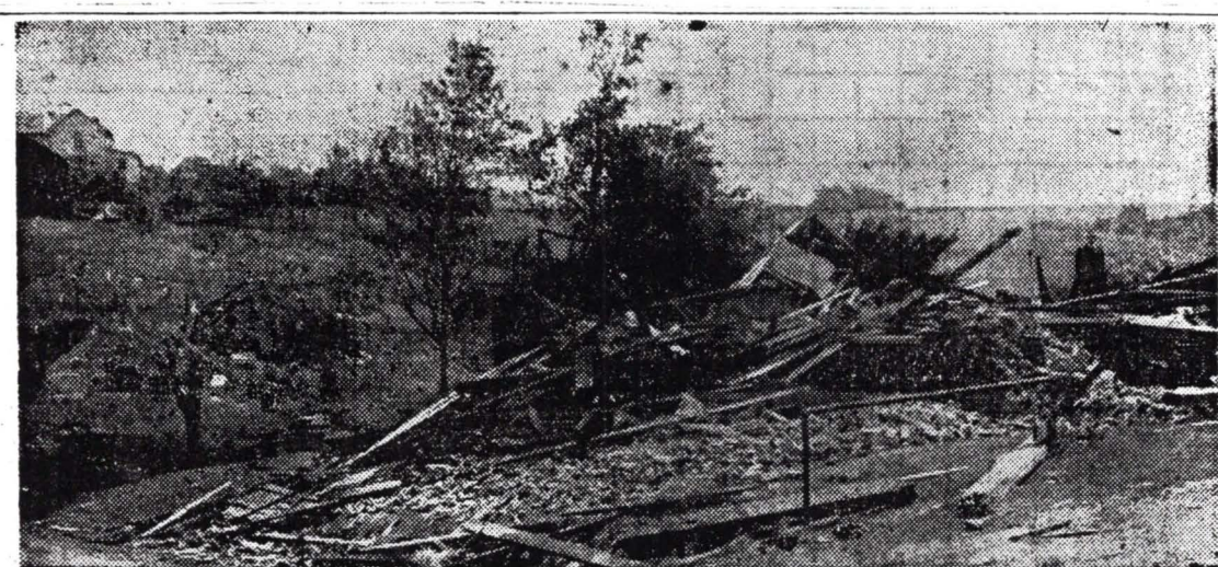
The Mt. Zion Baptist Church, a brick structure, went the way of all other buildings in the path of the cyclone. Here is a picture of the wreckage.
