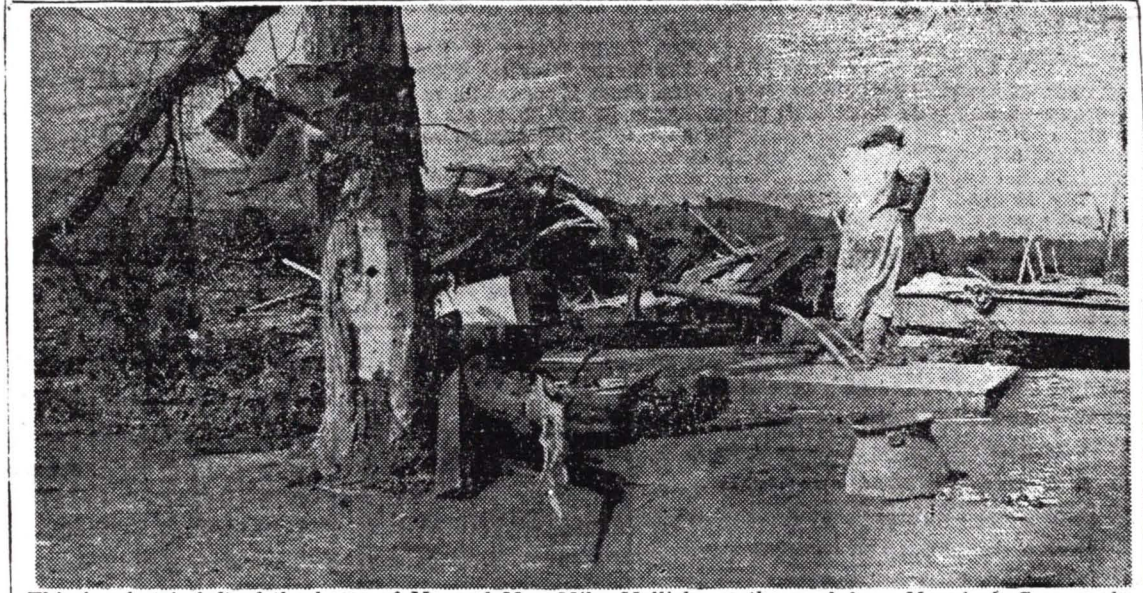
This is what is left of the home of Mr. and Mrs. Mike Mellish, on the road from Moredock Crossroads to Pollock Mill. Mrs. Mellish said that she and her husband sat in the house while the building blew away, and were only slightly injured. The kitchen blew away from around them and they went to the living room. In a few minutes the rest of the house blew away, leaving them standing on the ground floor. "We were blown some distance," Mrs. Mellish said. "I suffered some bad bruises and my husband has a cut above his right eye." Mrs. Mellish was in tears, because she had lost everything she had.
